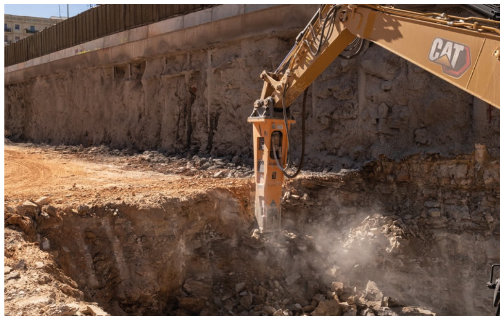
One of the two HP 5000 coupled with CAT 330 excavators complete the fleet at the Andria construction site
