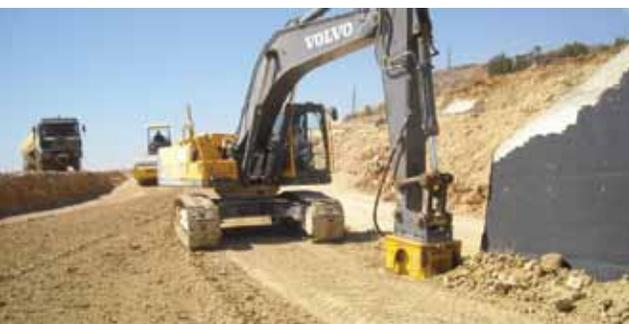
Since 2009, the Lebanese company Hourieh Enterprises has been using an Indeco IHC 200 compactor mounted on a Volvo 2006. The compaction plate is used for flattening the surfaces of motorways and main roads, and for compacting trenches and drains. In the photo: compacting soil on a slope by the roadside. ■
