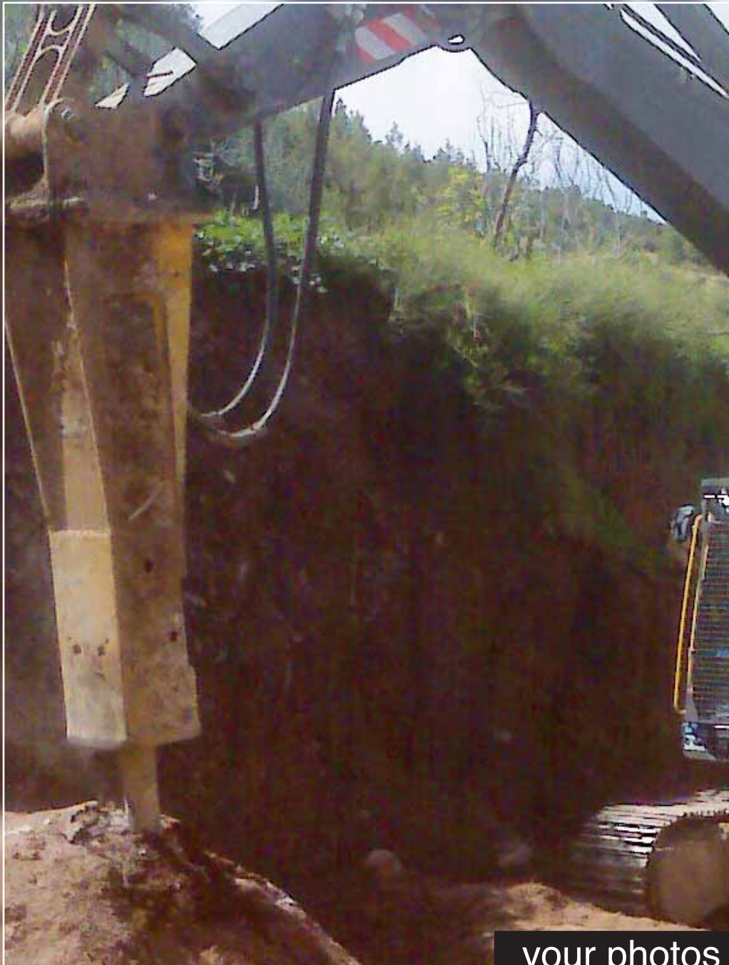
An Indeco HP 3500 working on conduits in Morocco's Atlas mountains. Photo by Souldi Abderrahmane.
