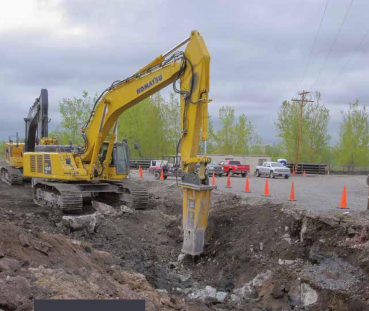
**For the demolition job, LP Ciminelli used five Indeco breakers – two HP 8000s, two HP 13001s and an HP 16000**
