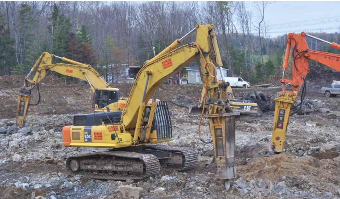
**Just outside Quebec City near the town of Levis, three Indeco breakers are digging an artificial lake.**
