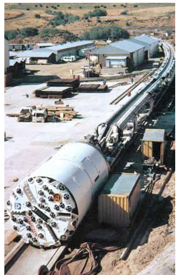
TBM used for Lesotho Highlands water supply project (Tambo_CC BY-SA)
