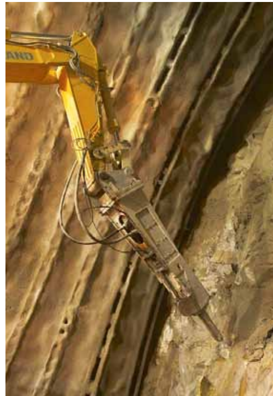
Indeco Breaker on excavation face
