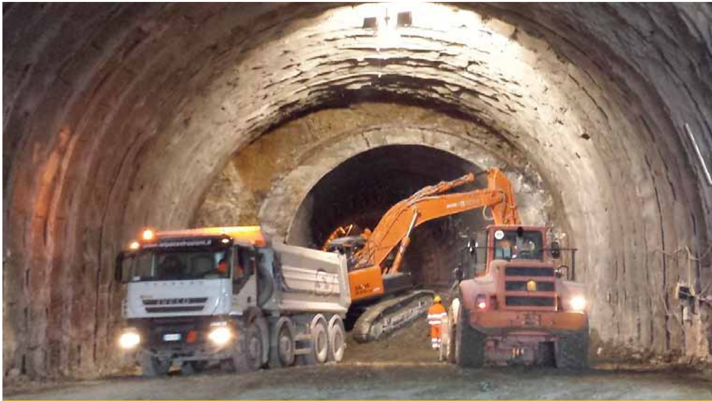
Partial excavation of tunnel enlargement, A3 SARC Normanno, HP 7000 on Hitachi 470
